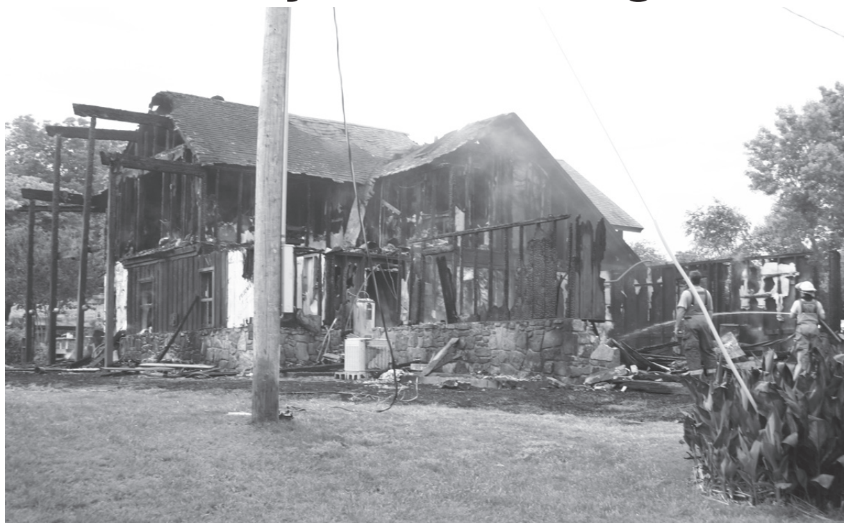
Local residents Jimmy and Violet Henderson lost their home to an early morning fire last Wednesday. The family home was destroyed by flames and smoke and water damage. An investigation is ongoing at this time.
